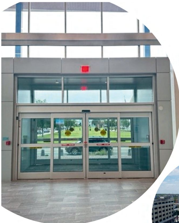
Pearl Street Exit
