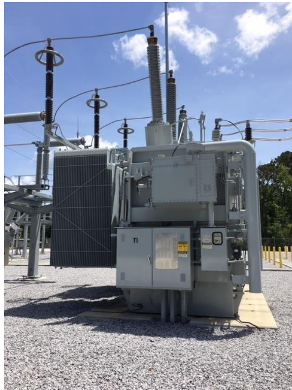
230kV/26kV Transformer
