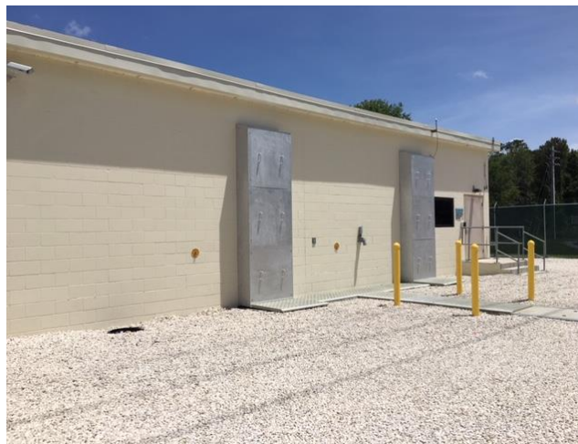
CONTROL HOUSE (OUTSIDE VIEW)
