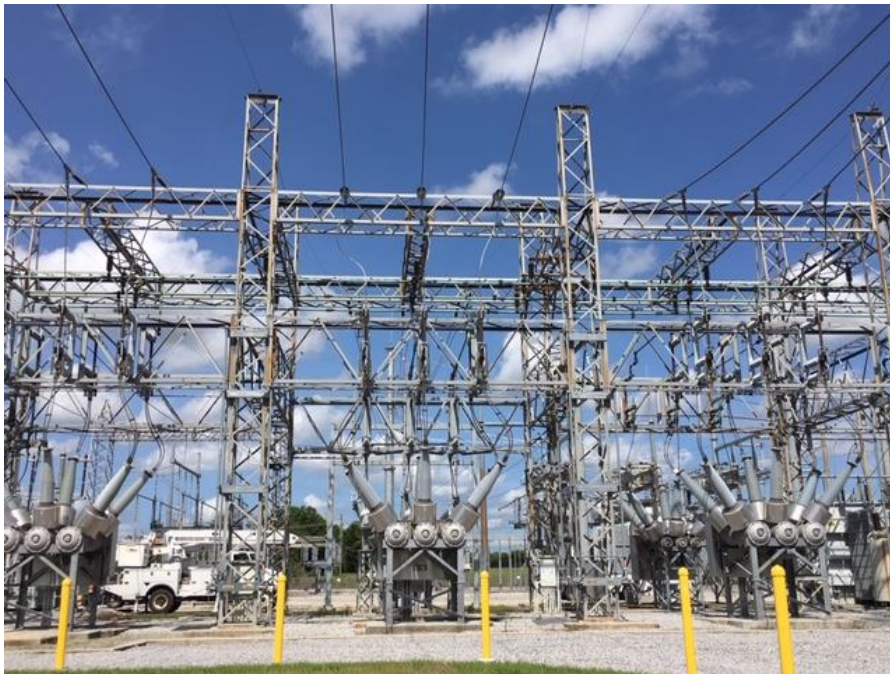
High Profile Lattice Steel Design
