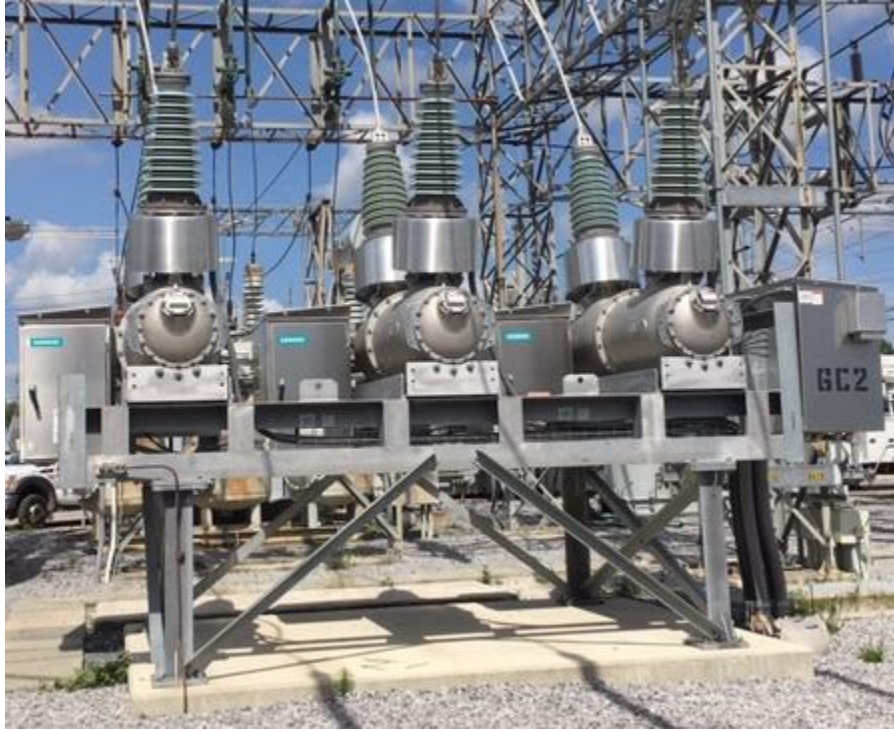
ZERO CROSSING CIRCUIT BREAKER DETAIL
