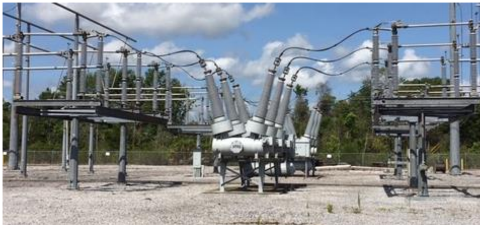
230KV CIRCUIT BREAKER DETAIL
