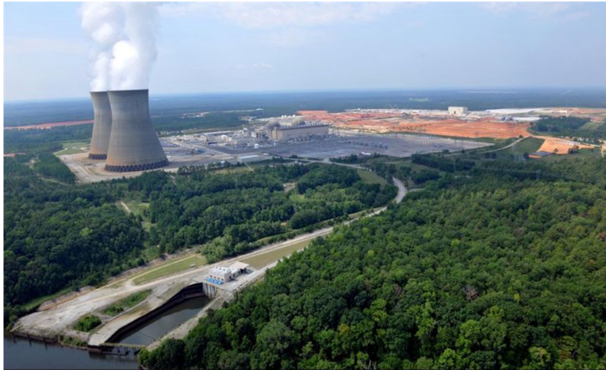
Aerial photograph of Vogtle site, with Vogtle 1 and 2 operating units to the left and Vogtle 3 and 4 construction site to the right. August 11, 2011 © 2011 Southern Company, Inc. All rights reserved.
