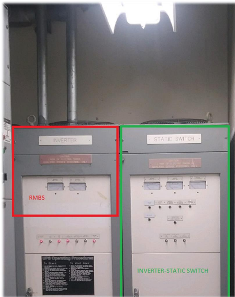
Location for New RMBS and Inverter-Static Switch.
