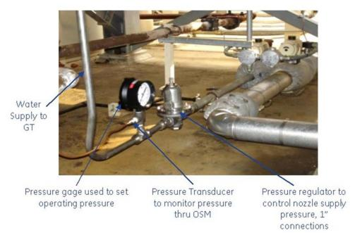
Figure 4: External changes to the water wash system
