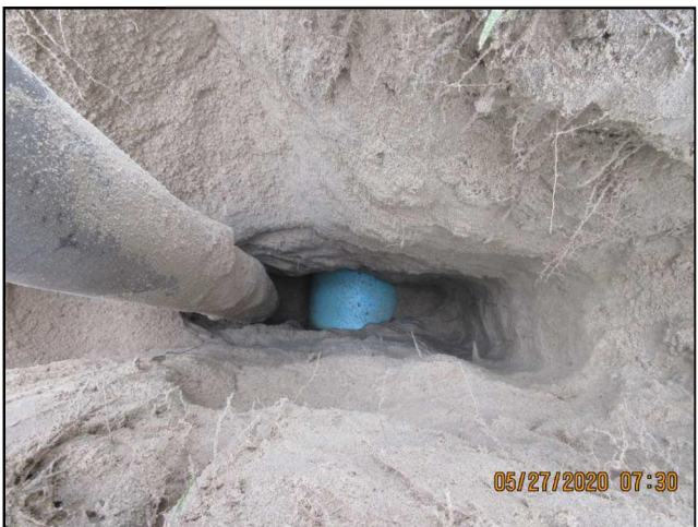
PICTURE DESCRIPTION: (Left) 12" Water Main 12.1' East of edge of pavement @ 4.98'. (Right) 20" Concrete pipe 8.3' East of edge of pavement @ 2.95'.
