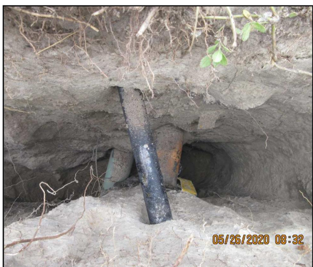
PICTURE DESCRIPTION: (Left) 6" AC Water Main (Abandoned) @ 3.38' and 0.5" Direct Buried Cable @ 2.09'. (Right) 2" Steel Pipe (Gas) @ 1.28', 4" PVC yellow Gas Main @ 2.99', and 4" Green PVC (unknown if gravity or FM) @ 3.92'.
