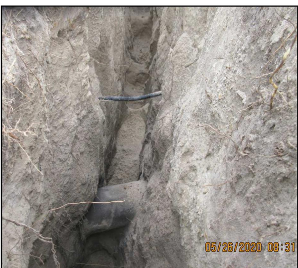
PICTURE DESCRIPTION: (Left) 6" AC Water Main (Abandoned) @ 3.38' and 0.5" Direct Buried Cable @ 2.09'. (Right) 2" Steel Pipe (Gas) @ 1.28', 4" PVC yellow Gas Main @ 2.99', and 4" Green PVC (unknown if gravity or FM) @ 3.92'.
