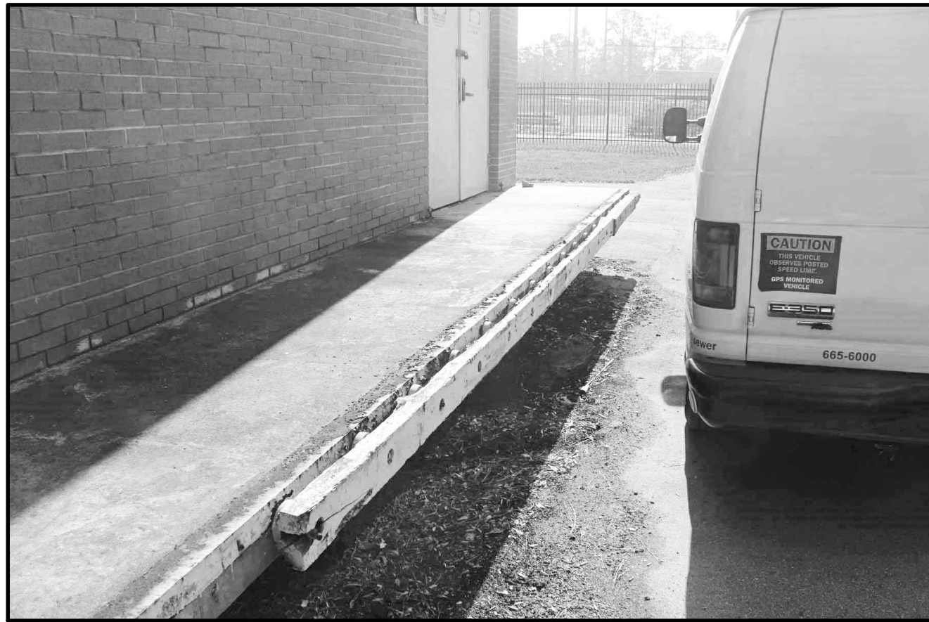
LOADING DOCK LOCATED ALONG FRONT OF BUILDING. REFURBISH NOSING, REPLACE DOCK BUMPER, INSTALL NEW ALUMINUM HANDRAIL AND TOEBOARD.
