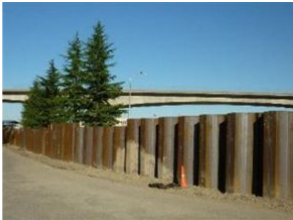
Tacoma WA Central Plant Flood Wall
