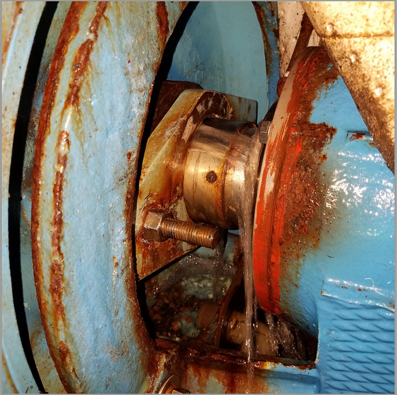
Image 2: N03 B River Water Booster Pump seals are leaking river water. The cantilevered impeller design typical for end suction centrifugal pumps will make this type of pump more prone to vibration and seal damage.
