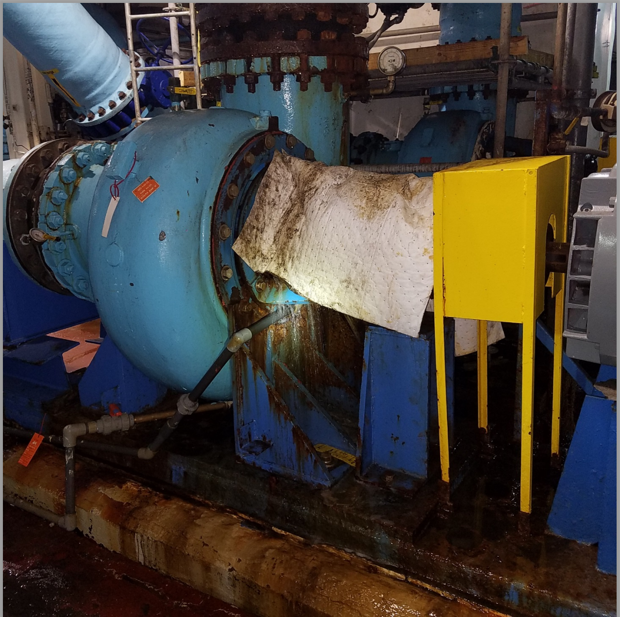
Image 1: Both N03 River Water Booster Pumps in parallel with B in the foreground and A in the background. Makeshift piping has been constructed in an attempt to stop flooding due to leaking seals.
