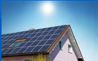
Rooftop PV (behind-the-meter)
