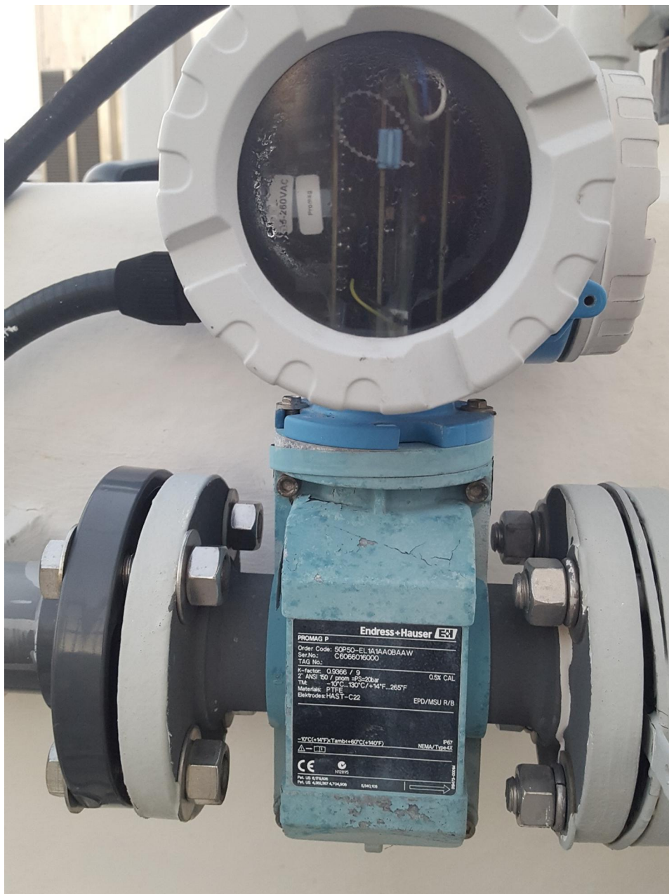
Unit 2B – display for flowmeter missing
