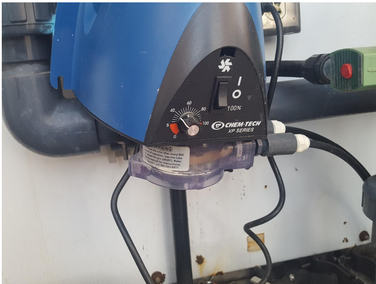
Unit 3A- Nutrient pump leaking
