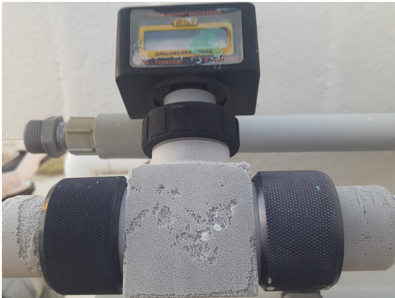
Unit 2B Non-working Flowmeter
