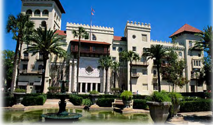
St. Johns County Courthouse
