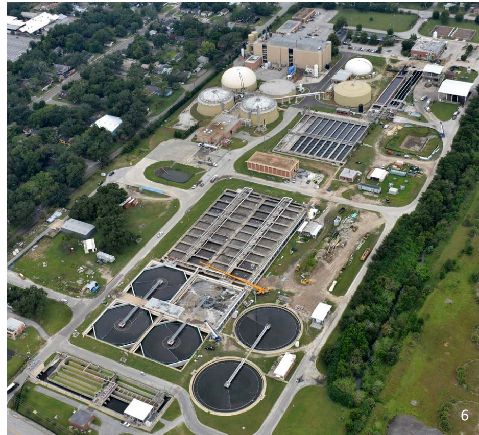
Buckman Wastewater Treatment Plant
