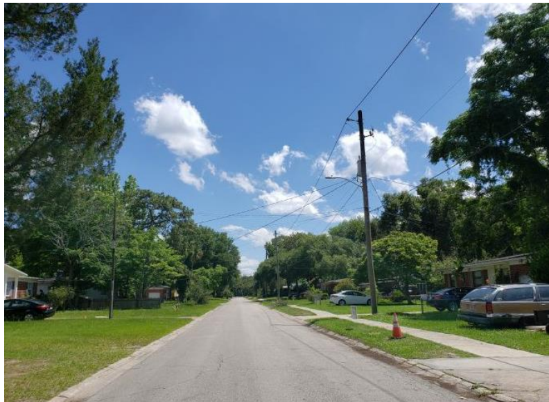
Figure 5-94: Eggleston Heights STPO Priority Area, Sprinkle Dr N Site Visit Photo
