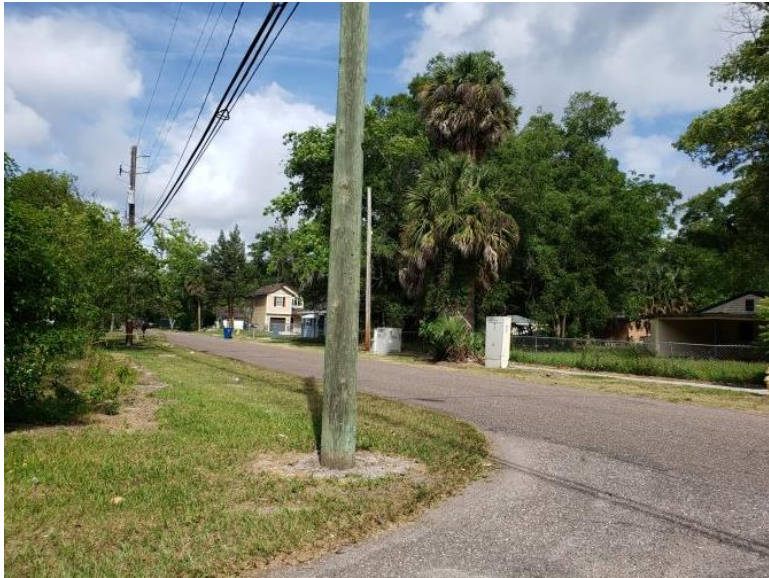
Figure 5-59: Riverview STPO Priority Area, Prospect St and 3rd Ave Intersection Site Visit Photo
