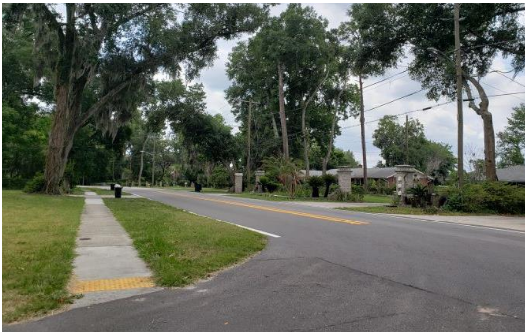
Figure 5-104: Lakeshore STPO Priority Area, Cedarwood Rd Site Visit Photo
