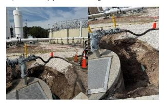
The site required significant dewatering to replace the pipe.
