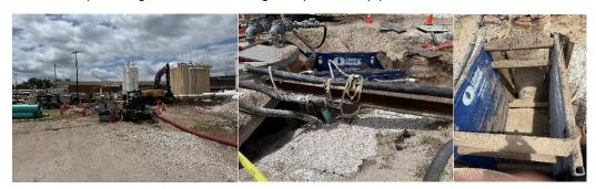
During construction another pipe was found to be collapsed. This pipe was not identified during CCTV inspection due to dirt in the pipe.
