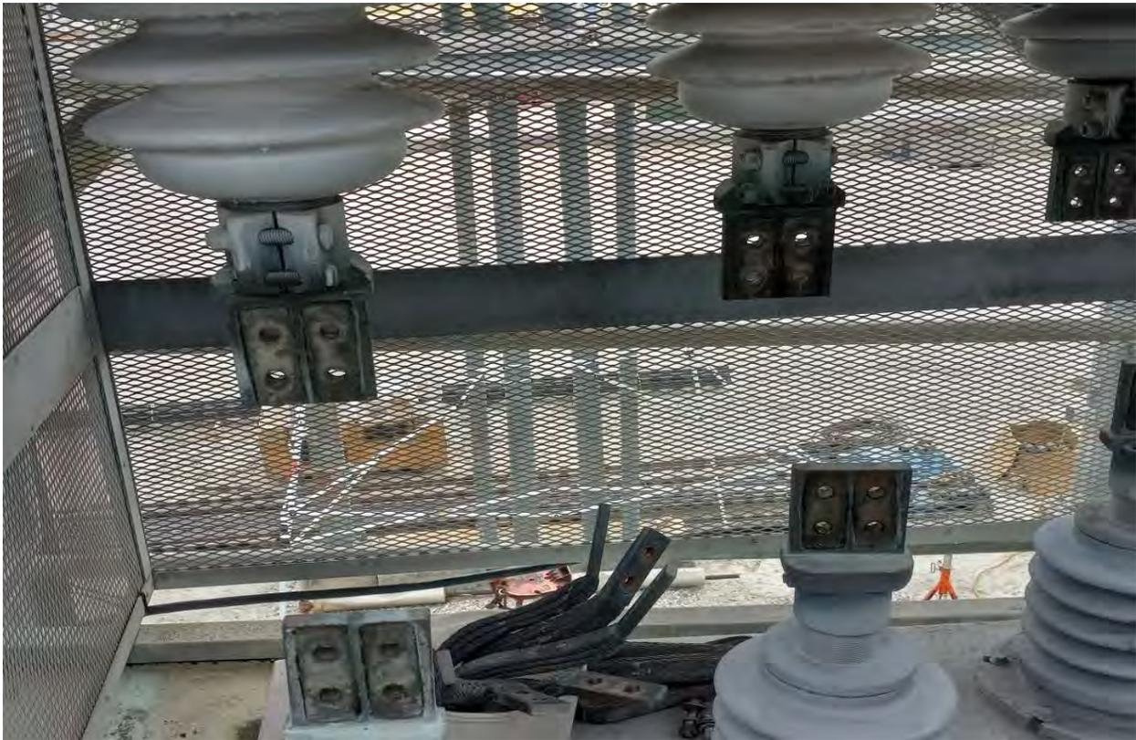
Top and Bottom Bushings at Generator and View of Eleven Inch Flex Links.
