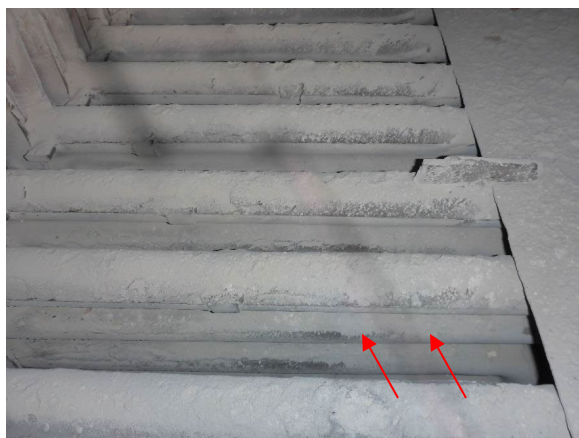
Buildup between tubes
