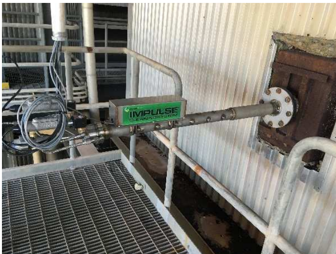
"Standard" Mounting Tube/Flange Part # 823-0128
