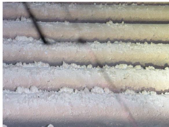
Scale buildup on tubes
