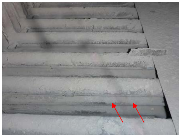
Buildup between tubes
