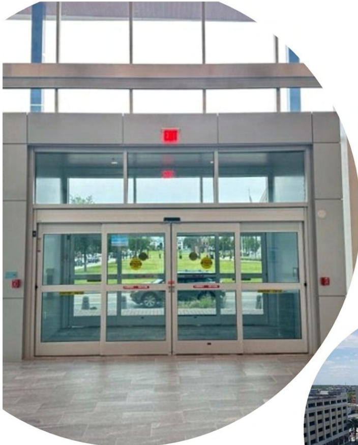
Pearl Street Exit
