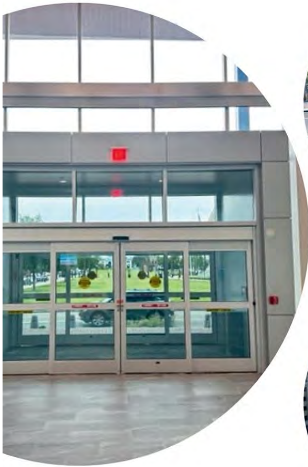
Pearl Street Exit
