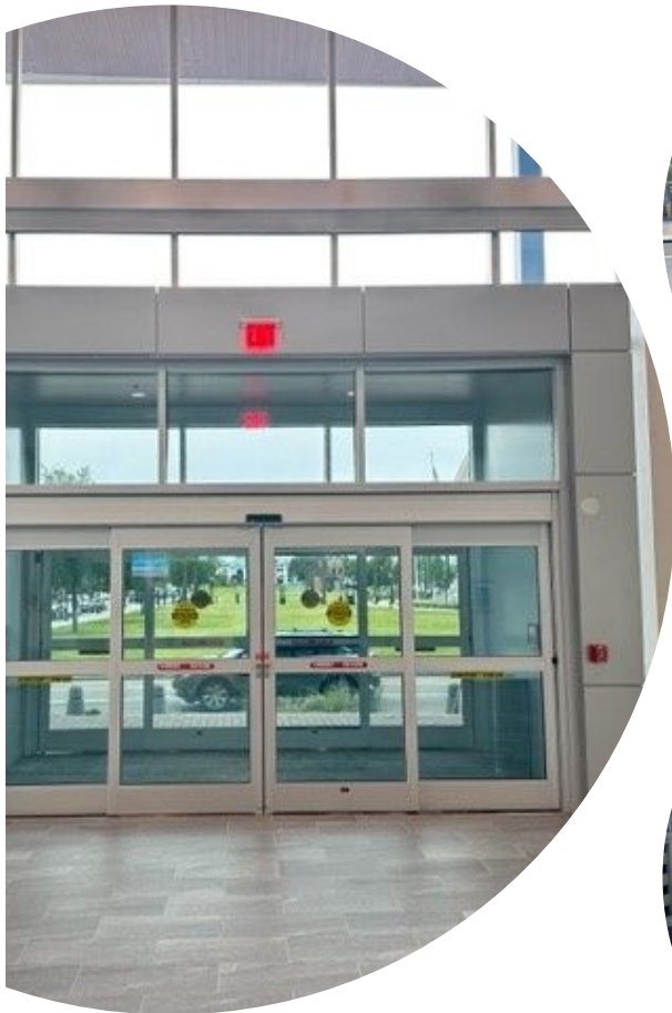
Pearl Street Exit
