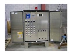
DESCRIPTION: Pump Station Electrical and Control Panel including (RTU) and Variable Frequency Drives (VFD). See Section 433 of the current JEA Standards for specifications and requirements.
