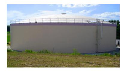
**DESCRIPTION:** Tanks are designed and built to AWWA and ACI standards and are made of low maintenance materials: concrete, stainless steel and fiberglass.
