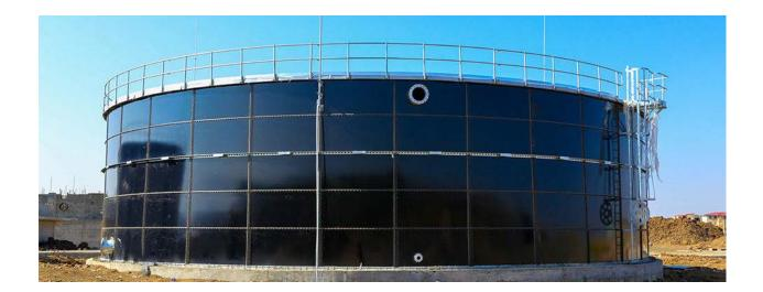
**DESCRIPTION:** This system is a storage tank made of sectional steel panels with glass molecularly bound (fused) to the steel surface. This provides a very durable, but flexible surface with excellent corrosion resistance, resulting in a tank, which can provide long life in a wide variety of applications.
