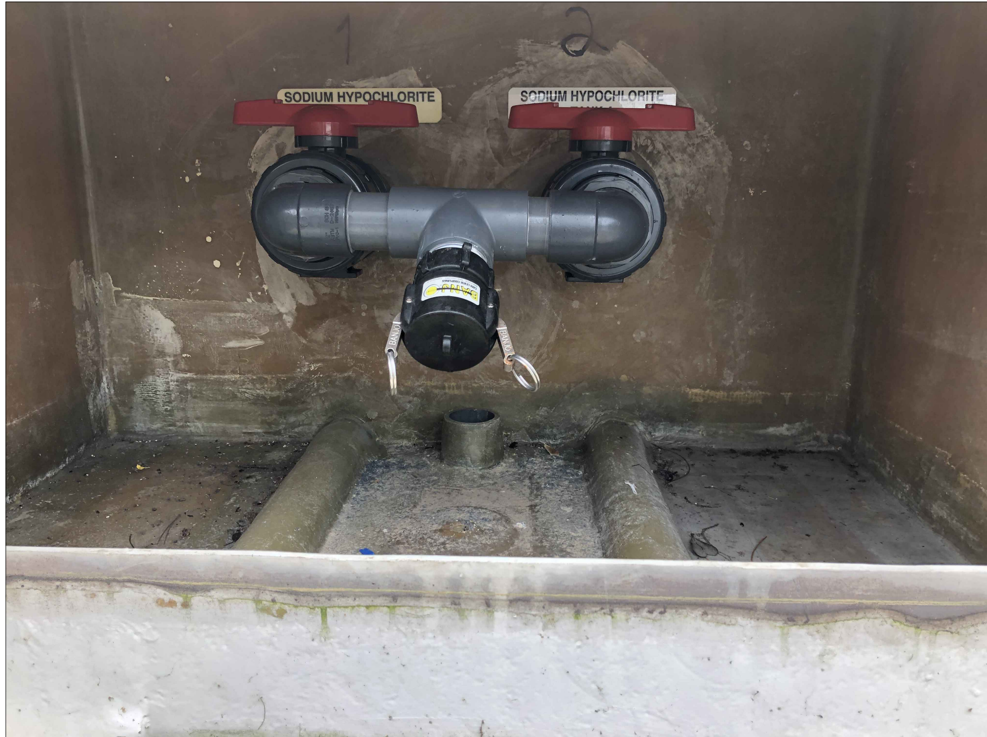
CHEMICAL FILL STATION PIPING
