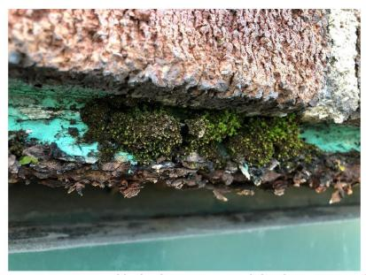
This moisture intrusion and lack of weeping capability has promoted organic growth and corrosion at the relief angle.
