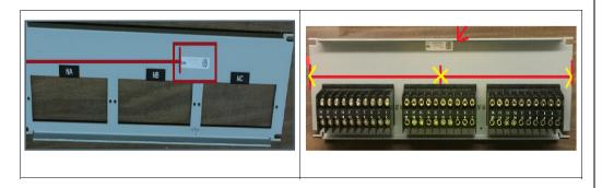
15. Internal test block nameplate shall be center aligned and 1/16" above it.
