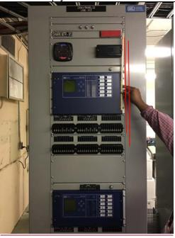
5. Controls Switch should be uniformly labelled with the Electroswitch Lockout Relay. Below is a picture of incorrect levelling:
