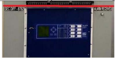
18. All front 19" plates should have bended edges. All plates should be mounted and centered with adjacent plate slots aligning properly.
