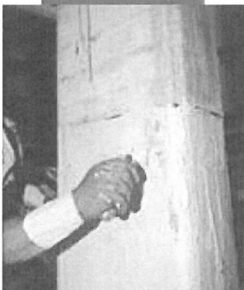
Levelling with Mapewrap 11 or Mapewrap 12
