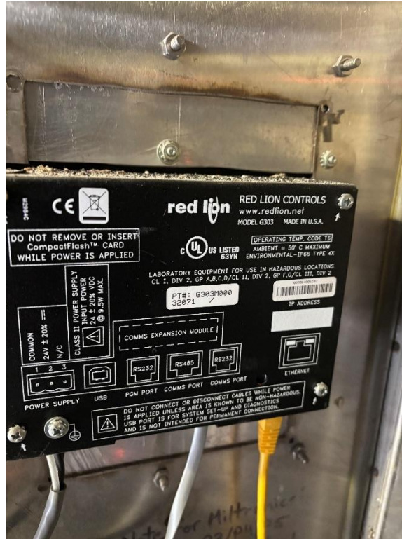
Figure 5: Existing RedLion Model G303 HMI
