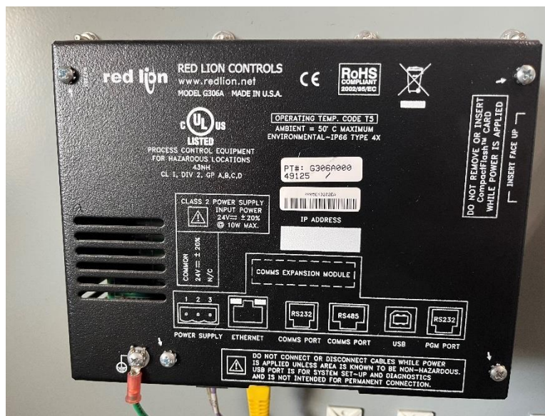
Figure 6: Existing RedLion Model G306A HMI
