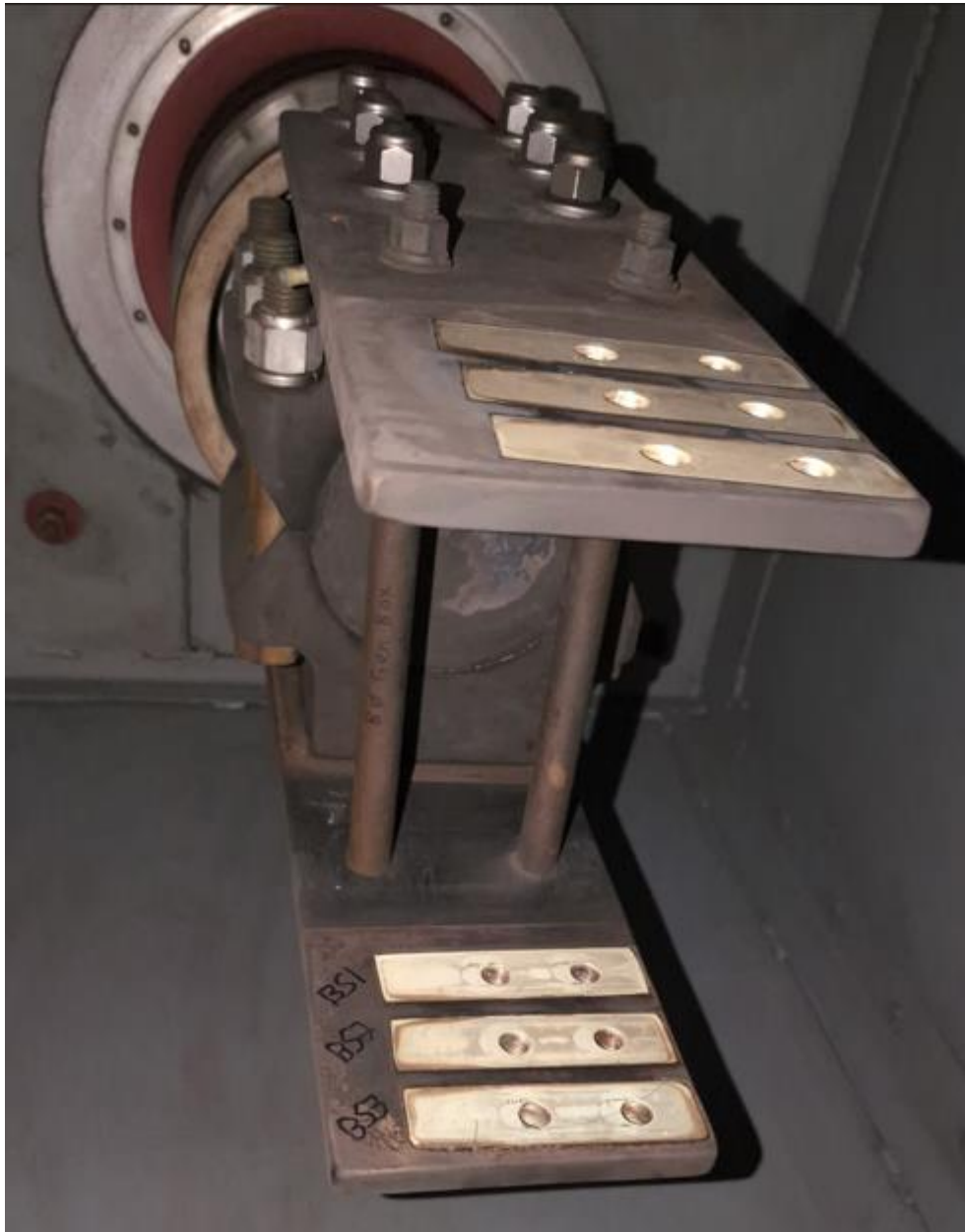
C Phase Generator Bushing Flex Links bolt to Inboard and Outboard Sides.
