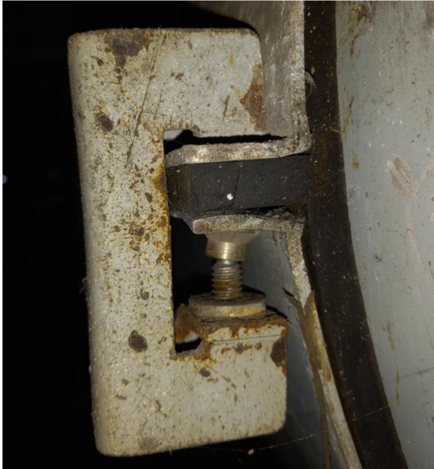
View of Bolting Clamp for N01 Enclosure Clamshells 2023.
