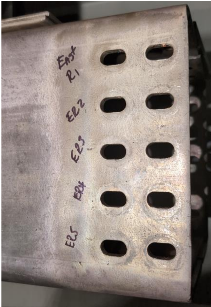
Neutral Bus Slotted Holes on Top, Bottom and both Sides.
