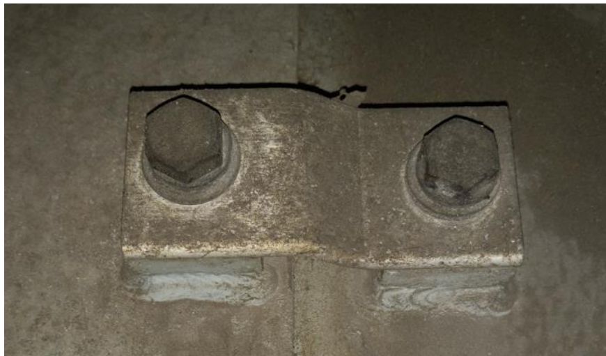
View of Bonding Linkage Between Enclosure and Clamshell 2023.
