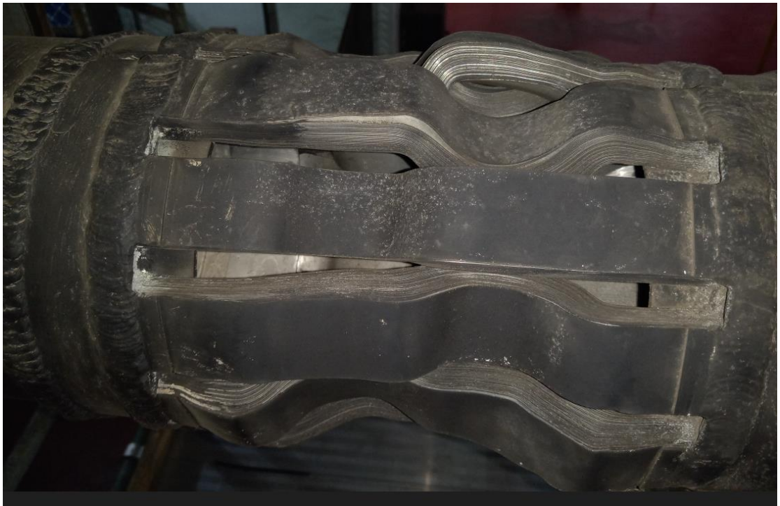
View of 12000A Main Bus Welded Connection 2023.
