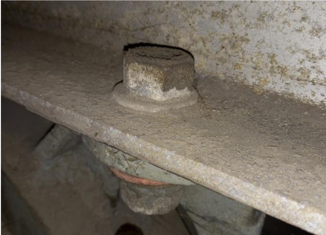
View from above of One Insulated Connection for Enclosure.
