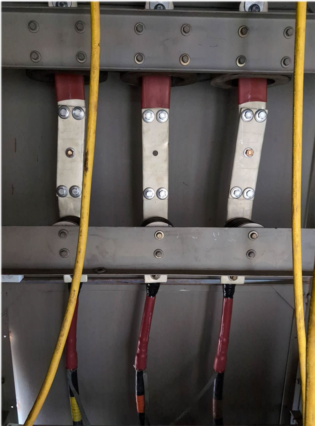
Bus Bar Below CT's Without Insulation Showing Bolting. Stainless Steel Hex Head Bolt, 1/2"-13 Thread Size, 2-1/4" Stainless Steel Hex Head Screw, 1/2"-13 Thread Size, 1" Qty:18 Attaches the bars to the insulators
