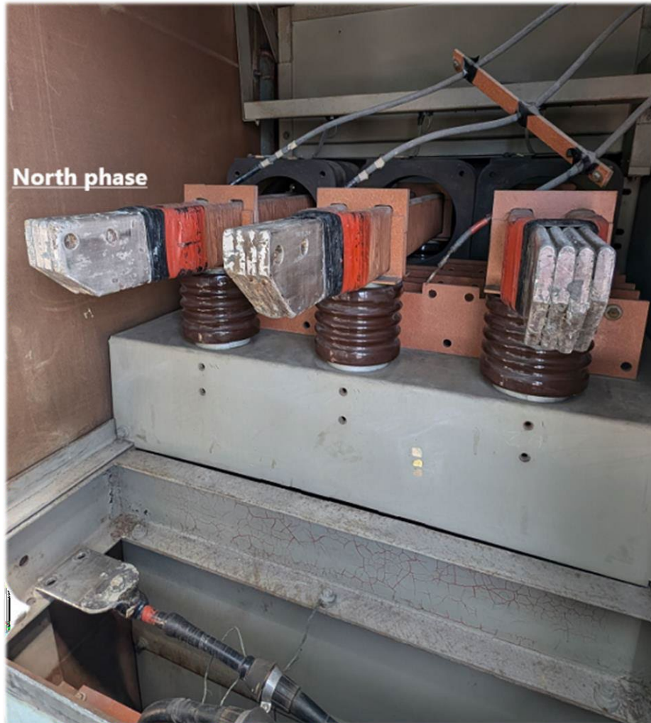
CT6 View of Bus Bar above Breaker. Looking East. Six Stainless Steel Hex Head Bolt, 1/2"-13 Thread Size, 5"
