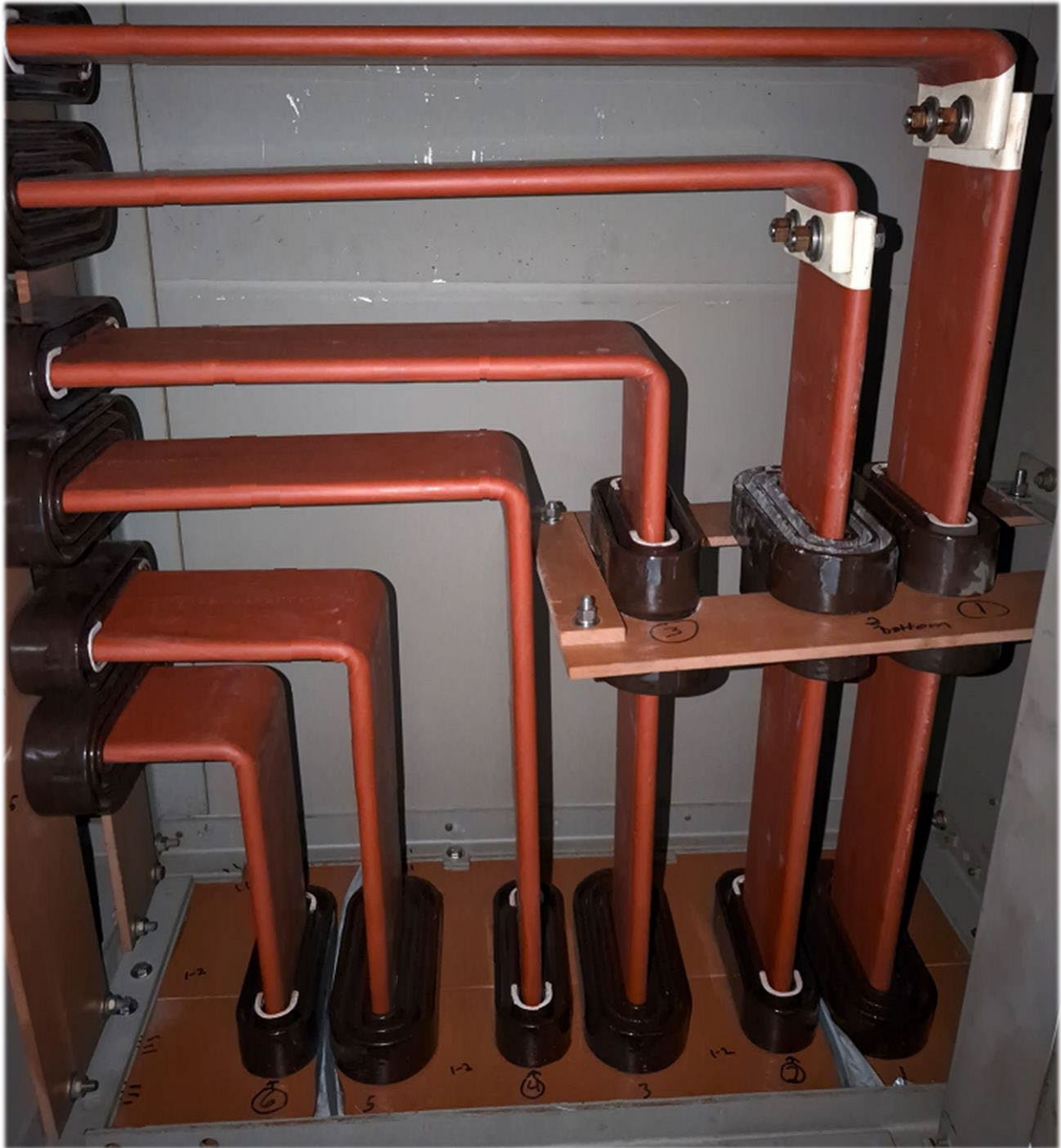
Leaving Transformer CT Compartment going to CT6's Refurbished PT Compartment.
