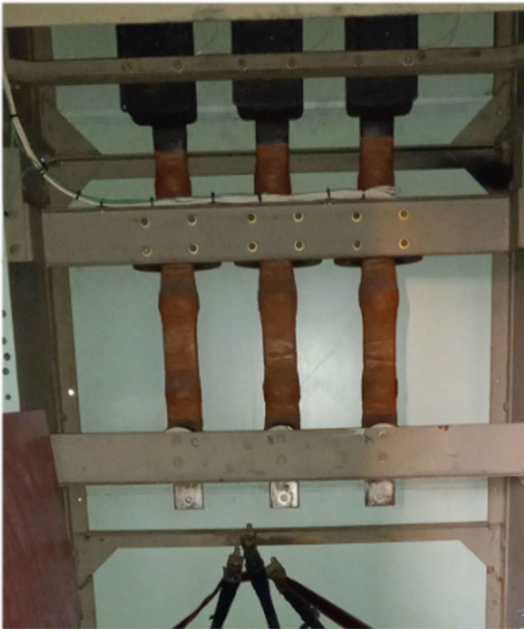
Transformer CT Compartment from Inside Switchgear.
