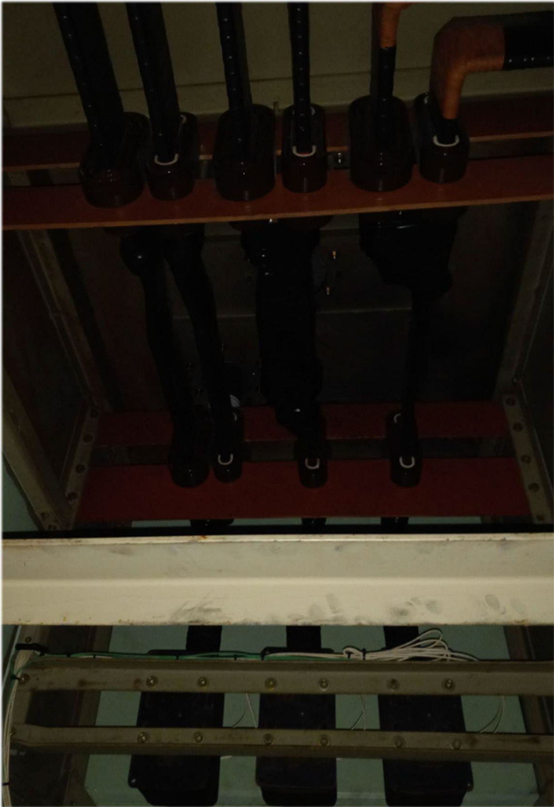
Transformer CT Compartment from Inside Switchgear.
