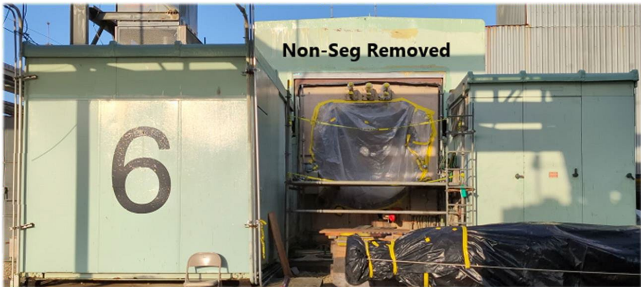
13.8 Switchgear on Left, Non-Seg Above Gen Removed, Excitation on Right.
