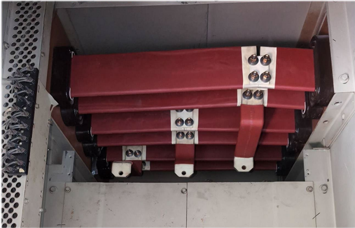
PT Compartment from Inside CT3's Refurbished Switchgear Showing Bolting. Bus Bar Connections: Stainless Steel Hex Head Bolt, 1/2"-13 Thread Size, 2-1/2" PT Connections: Stainless Steel Hex Head Bolt, 1/2"-13 Thread Size, 1"
