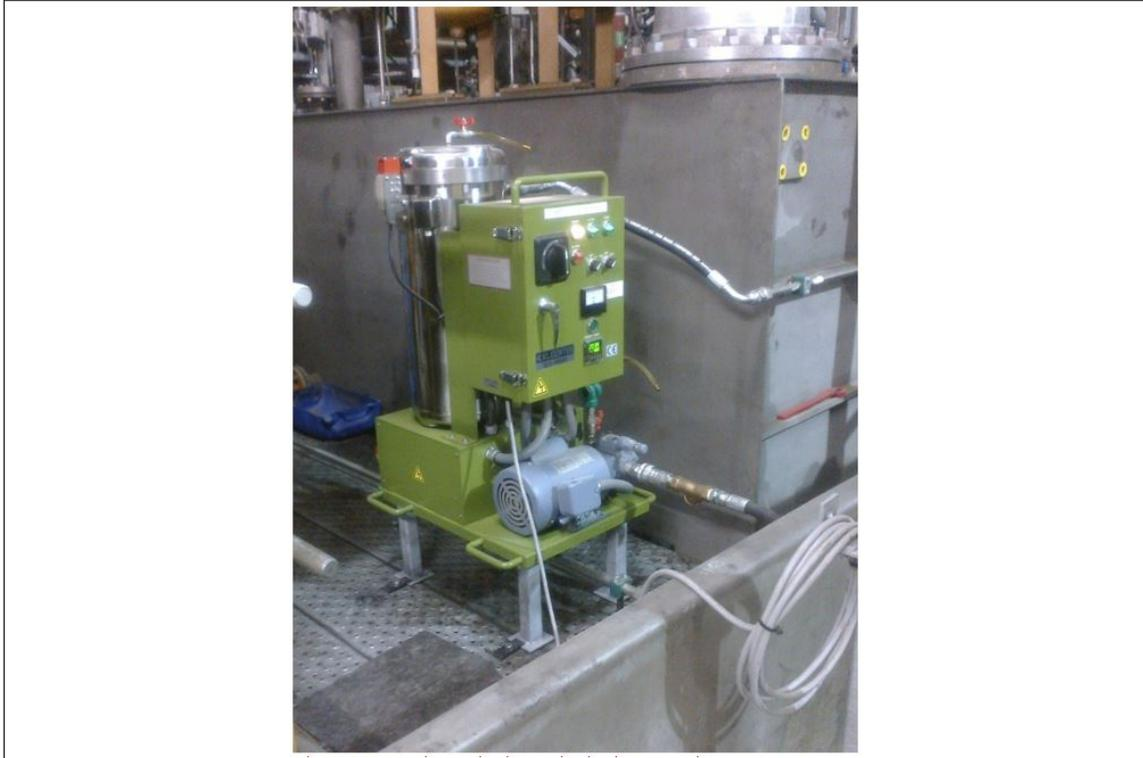
Fig. 4. Lube oil purifying skid inside containment area
