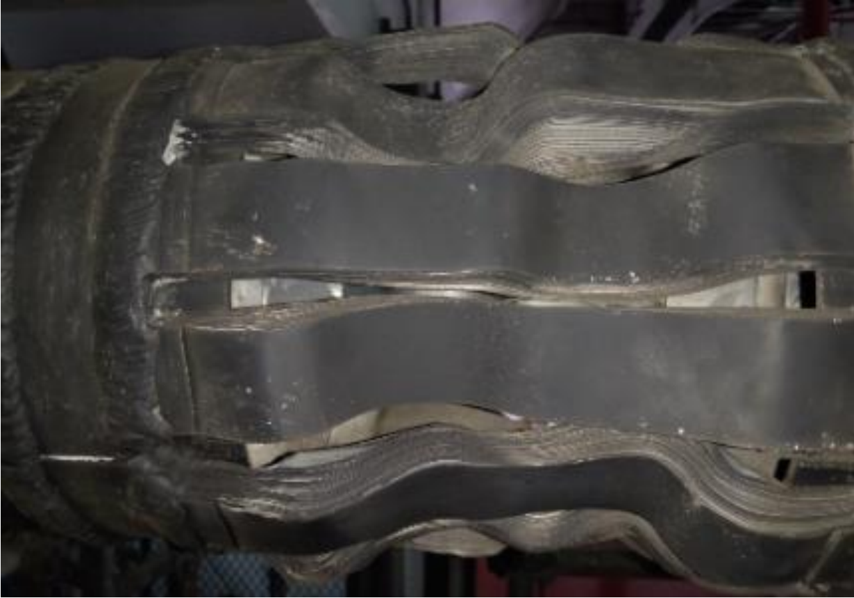
Figure 12, 13. 12,000A Welded Expansion Joint. No photo available for 1,200A Expansion Joint. They might not exist.
