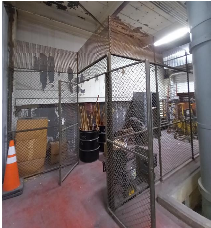
Metal Cage Behind IPB on Mezzanine – 10' Tall, 30' Length.
