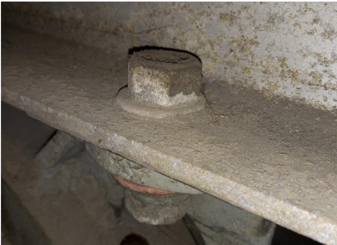
View from above of One Insulated Connection for Enclosure.
