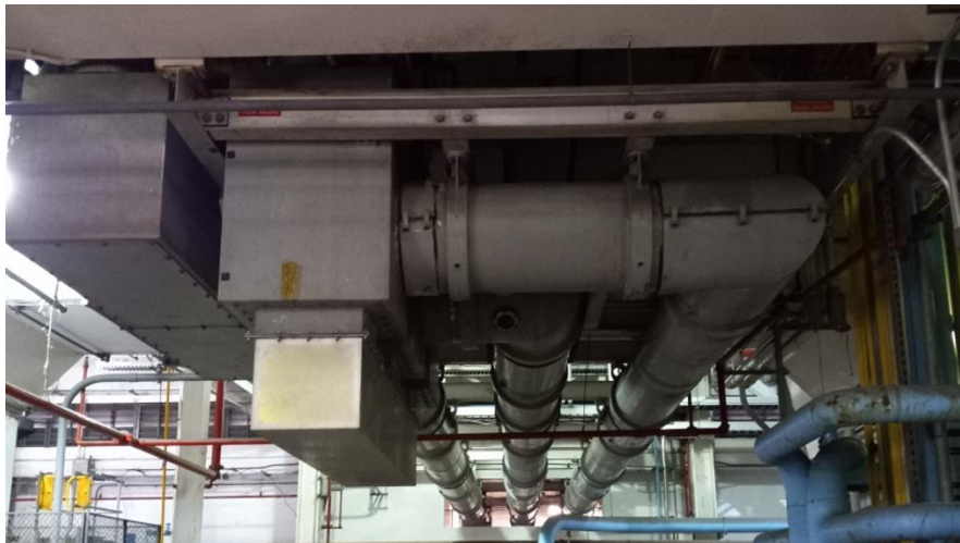
View of IPB on Mezzanine from below Generator 2023.
