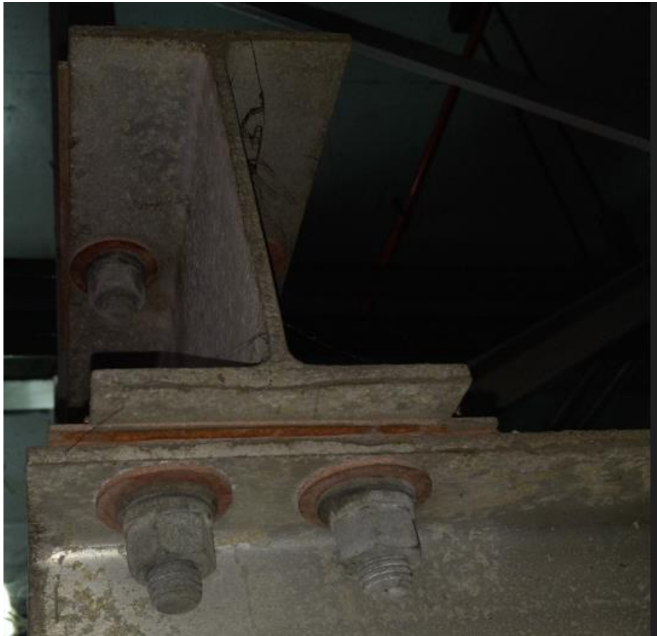
View of Insulation between Building Structure and IPB Bonding Structure.
