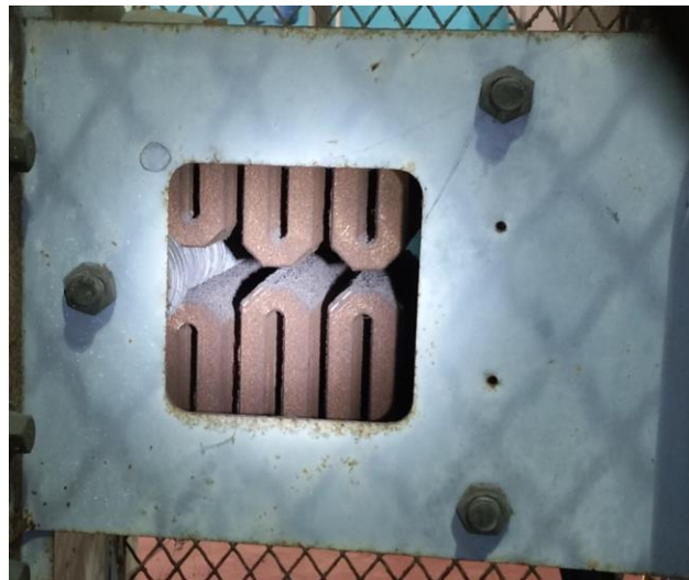
N01 NGR – Test resistance with calibrated (within 1 year) Ohm-meter.
