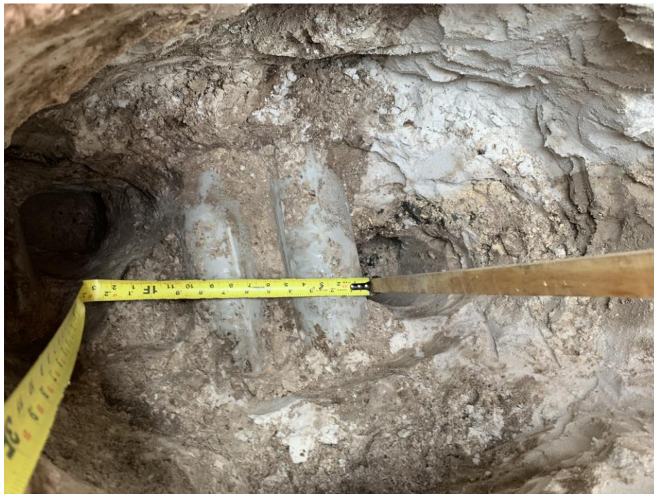
2-2" & 2-4" & 2-2" PVC COMMUNICATIONS CONDUITS
