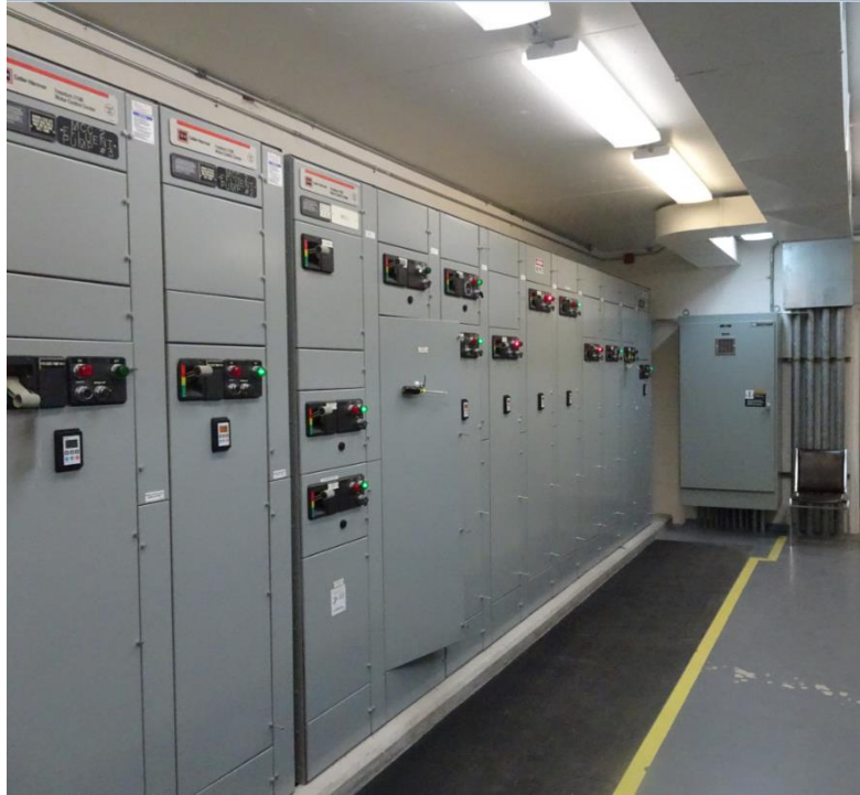
Left to Right: MCC-2, MCC-1, Automatic Transfer Switch
