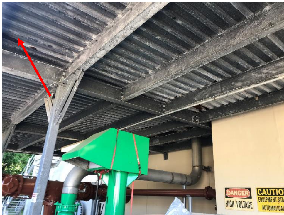
Photograph #12: View of canopy at SBR Basin. Note: Corrosion on underside of roof deck.
