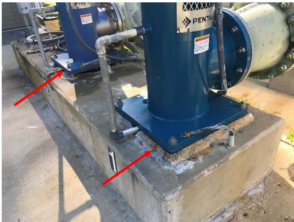
Photograph #20: View of effluent pumps at the UV Structure. Note: Missing grout under base plate, cracked and stained grout.
