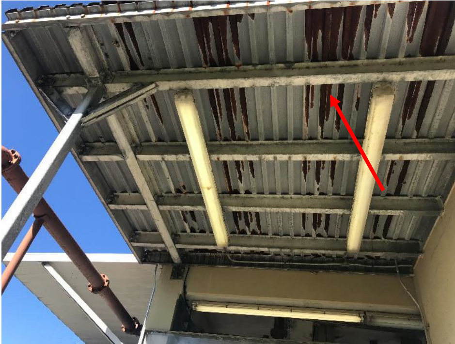
Photograph #7: View of roof framing and roof deck at Centrifuge Facility. Note: Corrosion visible on roof deck.
