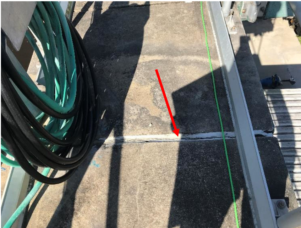
Photograph #18: View of walkway joint at SBR Basin. Note: Cracked and failing sealant.
