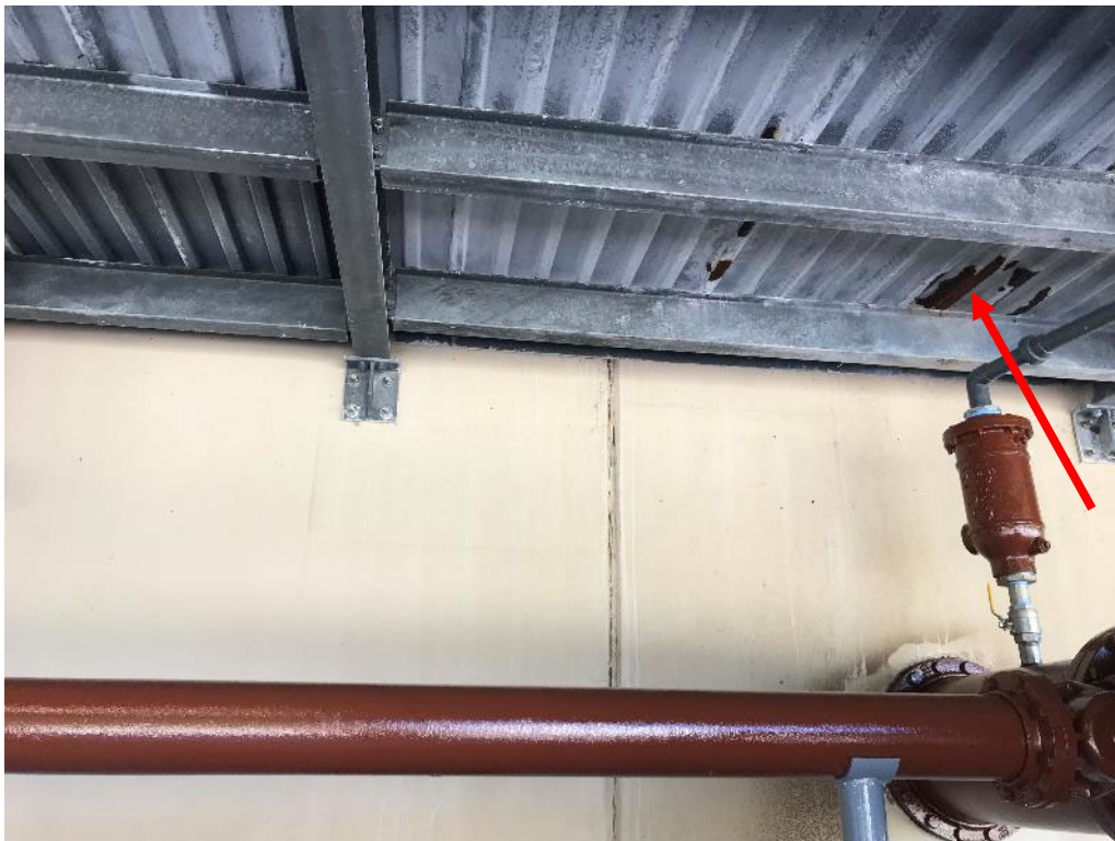
Photograph #13: View of canopy at SBR Basin. Note: Corrosion on underside of roof deck.
