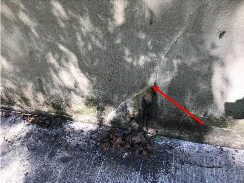
Photograph #15: View of typical cracking on walls at SBR Basin.
