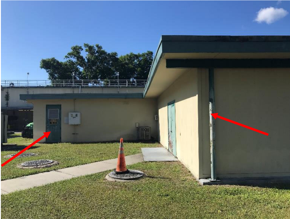
Photograph #25: View of Electrical Building. Note: Paint system failure at all doors and exterior columns and beams supporting the roof system.
