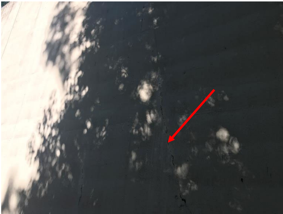
Photograph #16: View of typical cracking on walls at SBR Basin.
