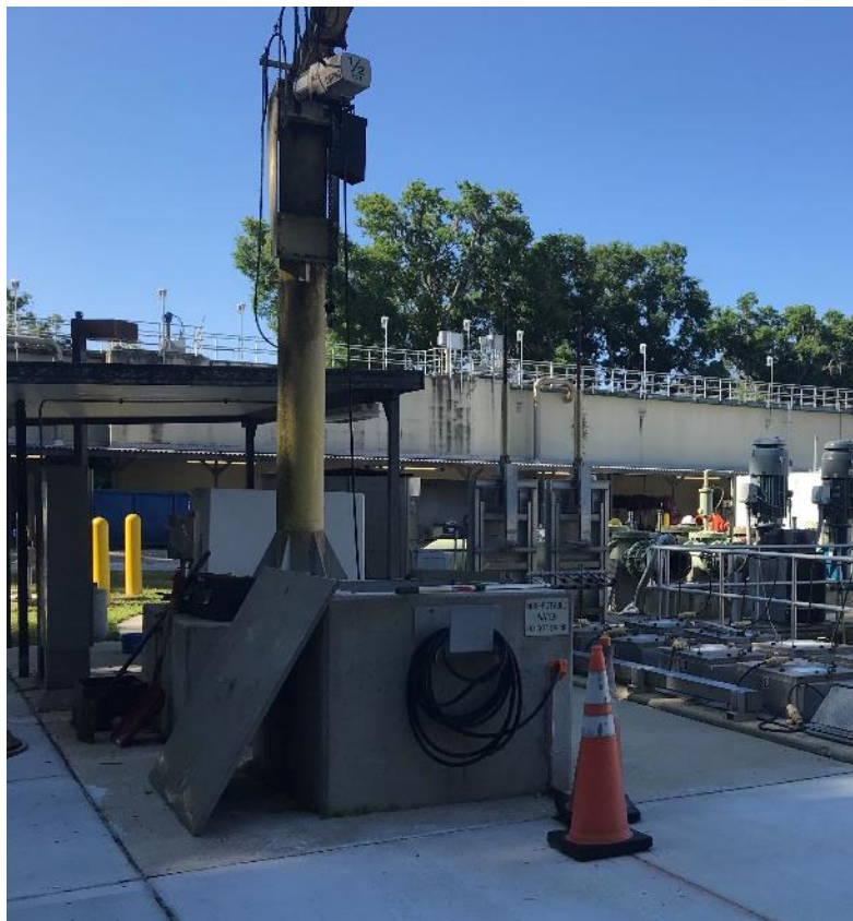
Photograph #22: View of davit crane at the UV Structure.
