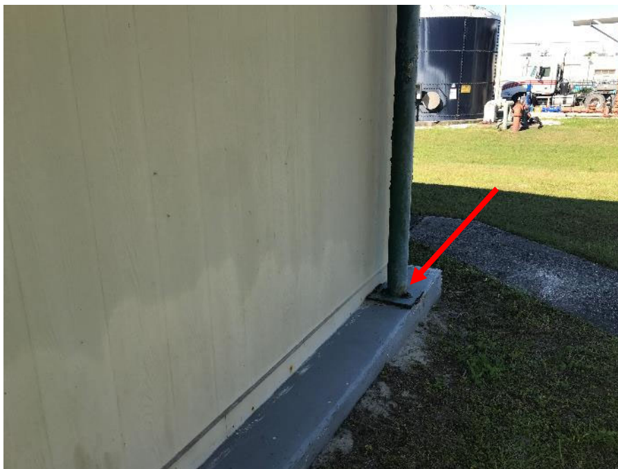
Photograph #26: View of Electrical Building. Note: Paint system failure at all doors and exterior columns and beams supporting the roof system.
