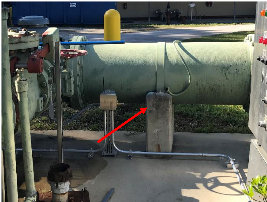
Photograph #21: View of effluent pipes at the UV Structure. Note: Cracked concrete pipe support.
