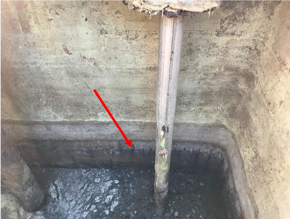
Photograph #1: View within pump station wet well. Note: Visible wall reinforcement and missing/failed coating system.
