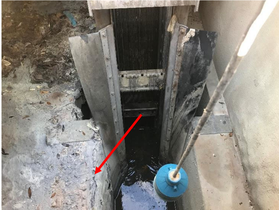
Photograph #3: View within screening channel. Note: Spalled concrete and failing coating system on channel wall.
