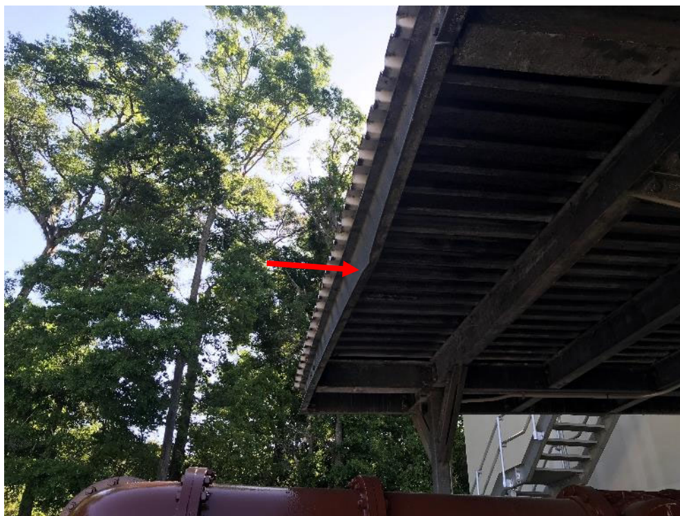
Photograph #14: View of canopy at SBR Basin. Note: Corrosion on underside of roof deck.
