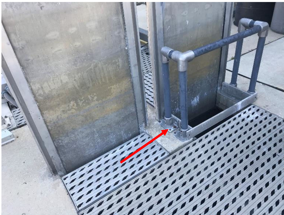
Photograph #19: View of gates and grating at UV Structure. Note: Corroded guardrail anchor bolts.
