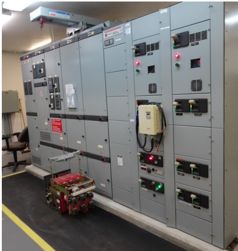
Left to Right: 480-volt Switchgear and MCC-3
