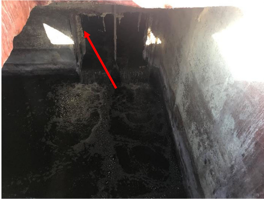
Photograph #5: View within pump station wet well. Note: Spalled and deteriorated concrete in vicinity of gate frames.
