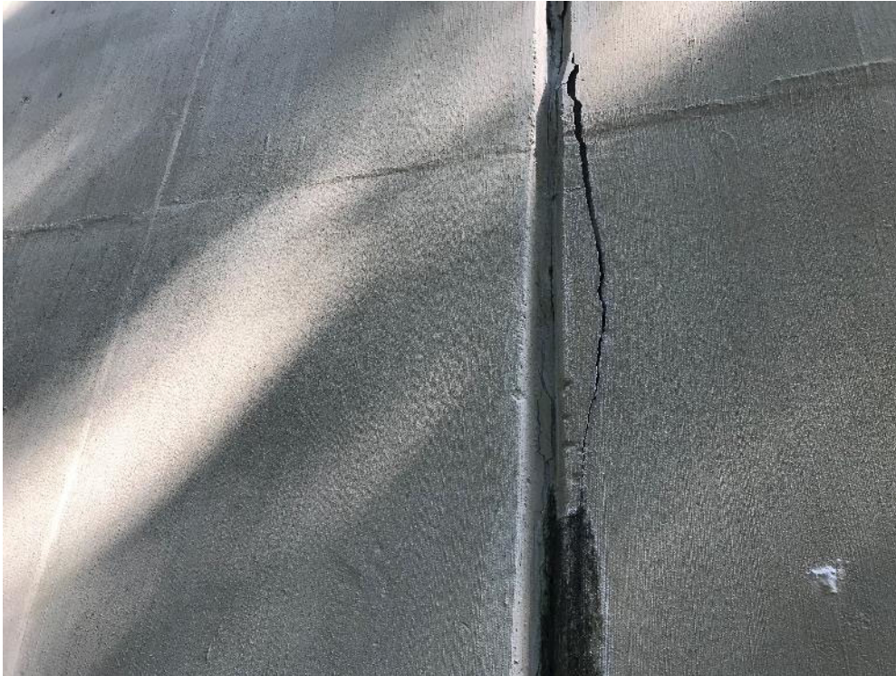
Photograph #17: View of spalling on walls at SBR Basin vertical joints.
