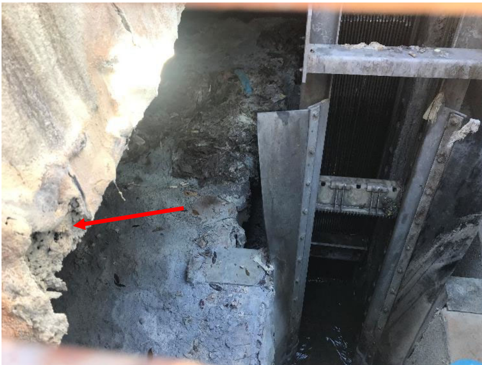
Photograph #4: View within screening channel. Note: Spalled and deteriorated concrete at concrete beam above channel.
