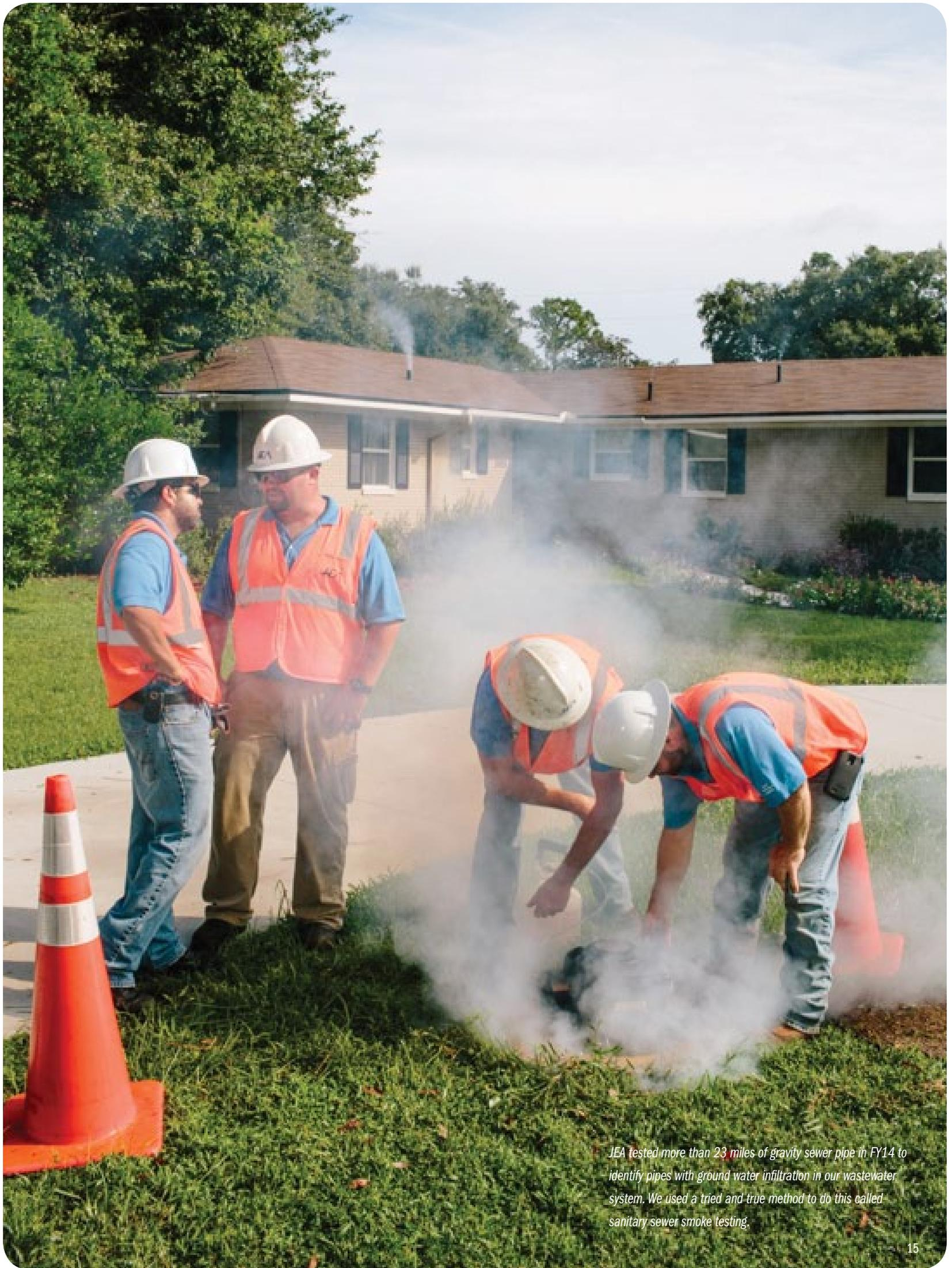
*JEA tested more than 23 miles of gravity sewer pipe in FY14 to identify pipes with ground water infiltration in our wastewater system. We used a tried and true method to do this called sanitary sewer smoke testing.*
