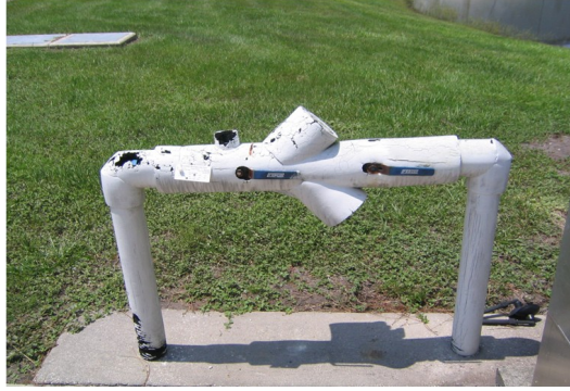
Reduced pressure principle backflow preventer
