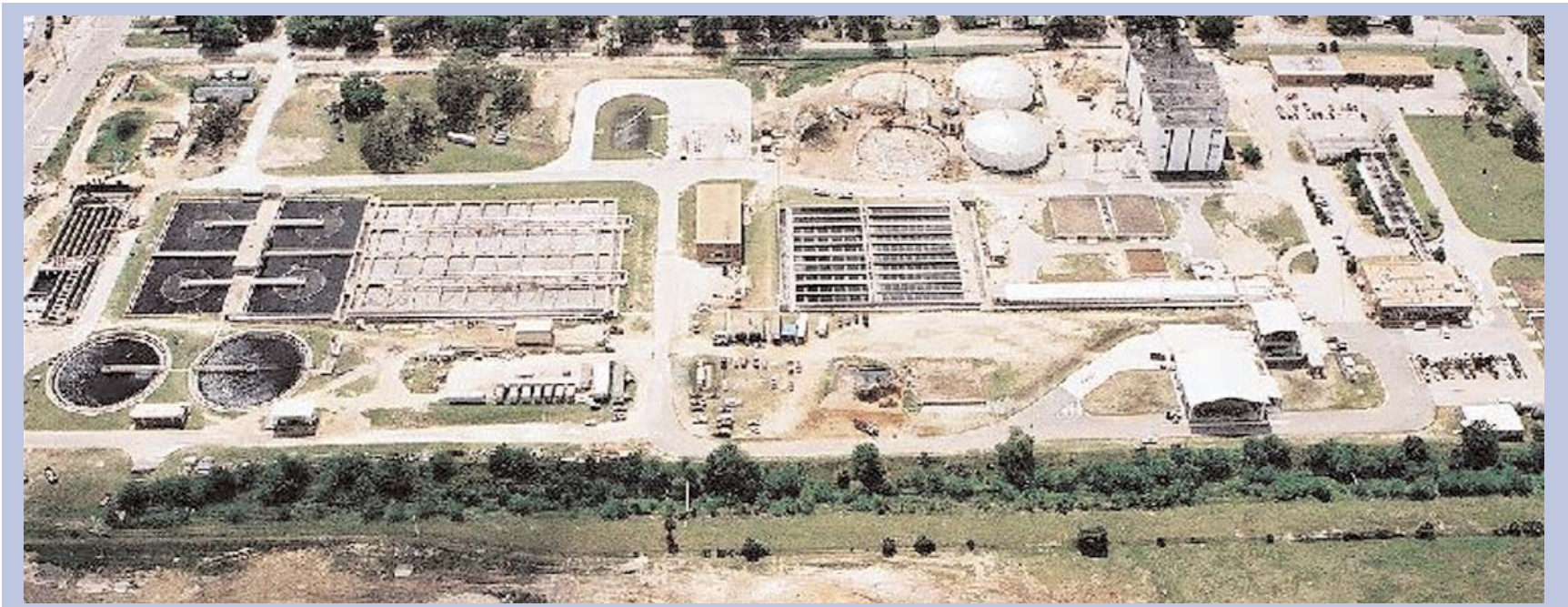
The Buckman WRF during construction of facility upgrades.
